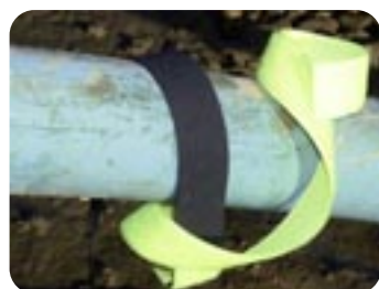
PLASTIC PIPE REPAIR
